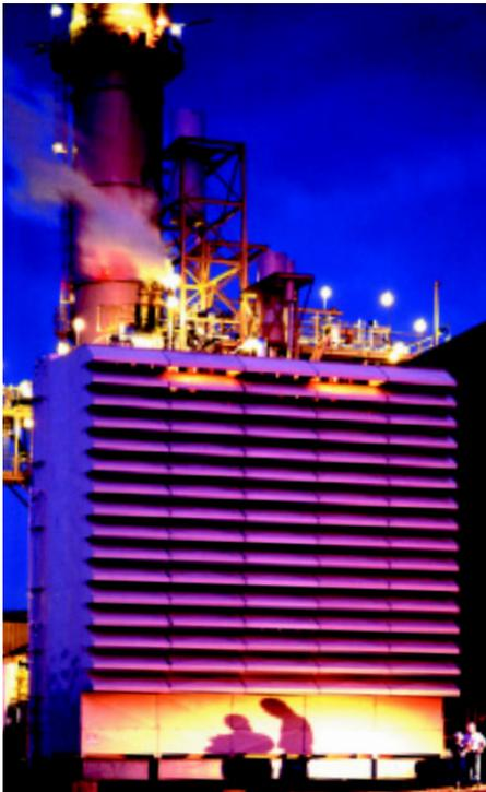
*The Donaldson evaporative cooler, positioned behind the GDX self-cleaning air filter, reduces inlet air temperature for a Siemens Westinghouse 501FC Gas Turbine near St. Paul, Minnesota, USA.*
